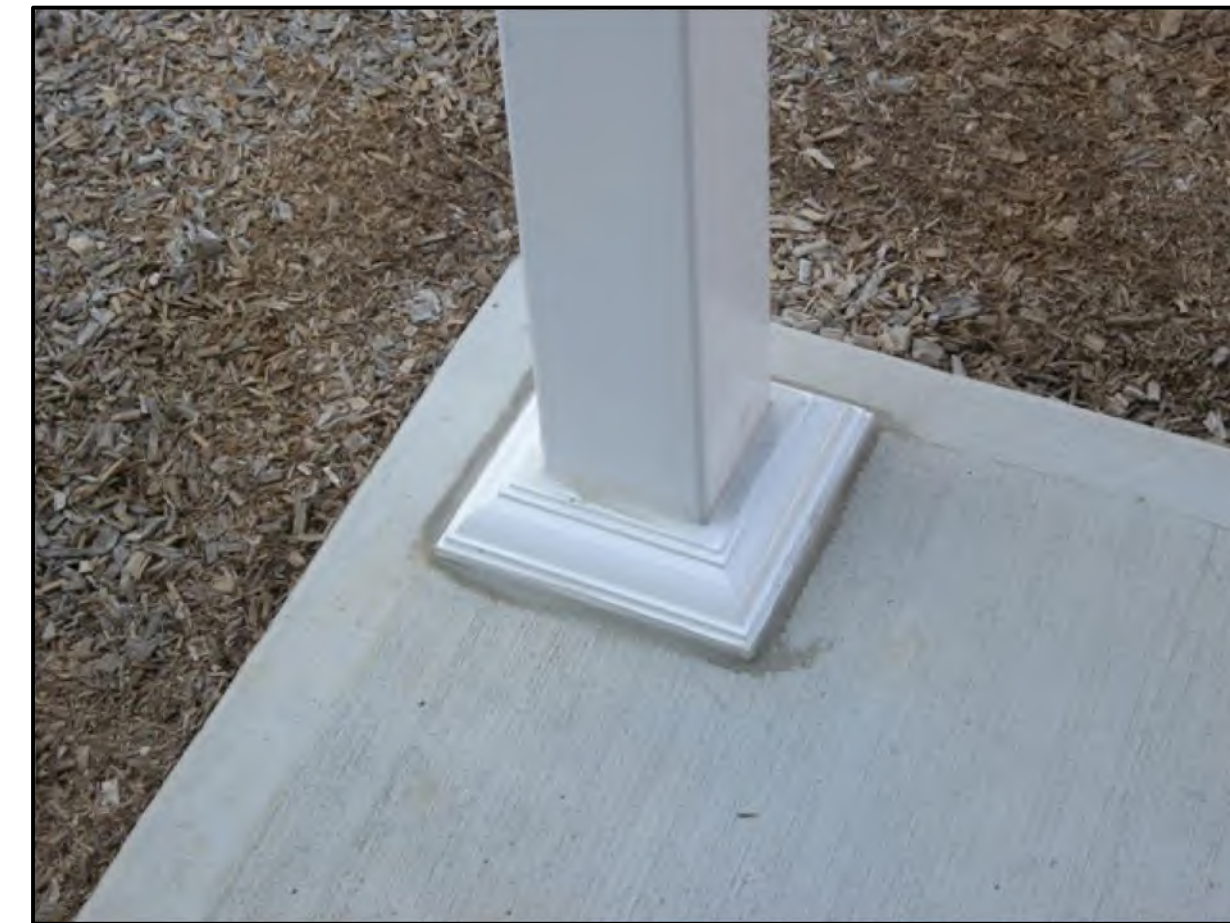
4 POST / CONCRETE PAD PICTURE
